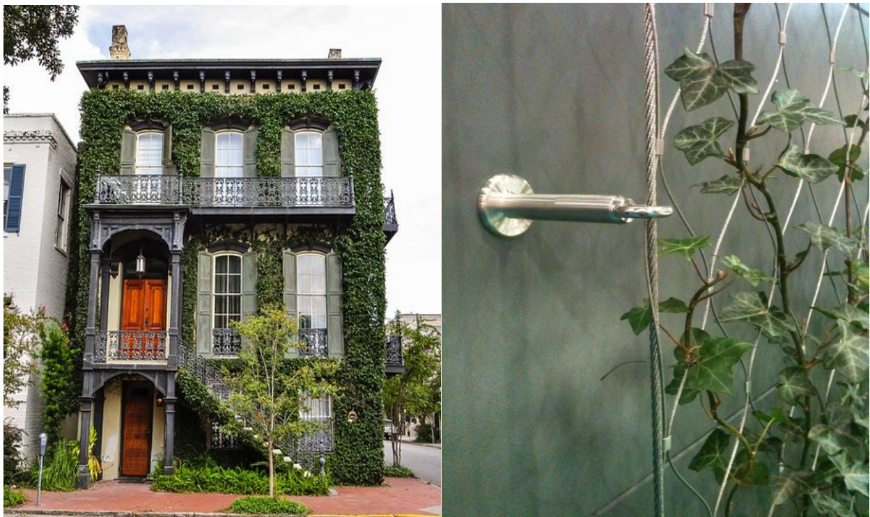
Figure 4. (Left) Direct system in Savannah, GA. (Right) Indirect System ( http://www.clairepotterdesign.com/ )
