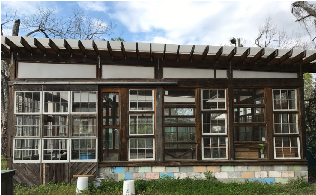
Figure 45. Southern Façade of the E. 34 Greenhouse
