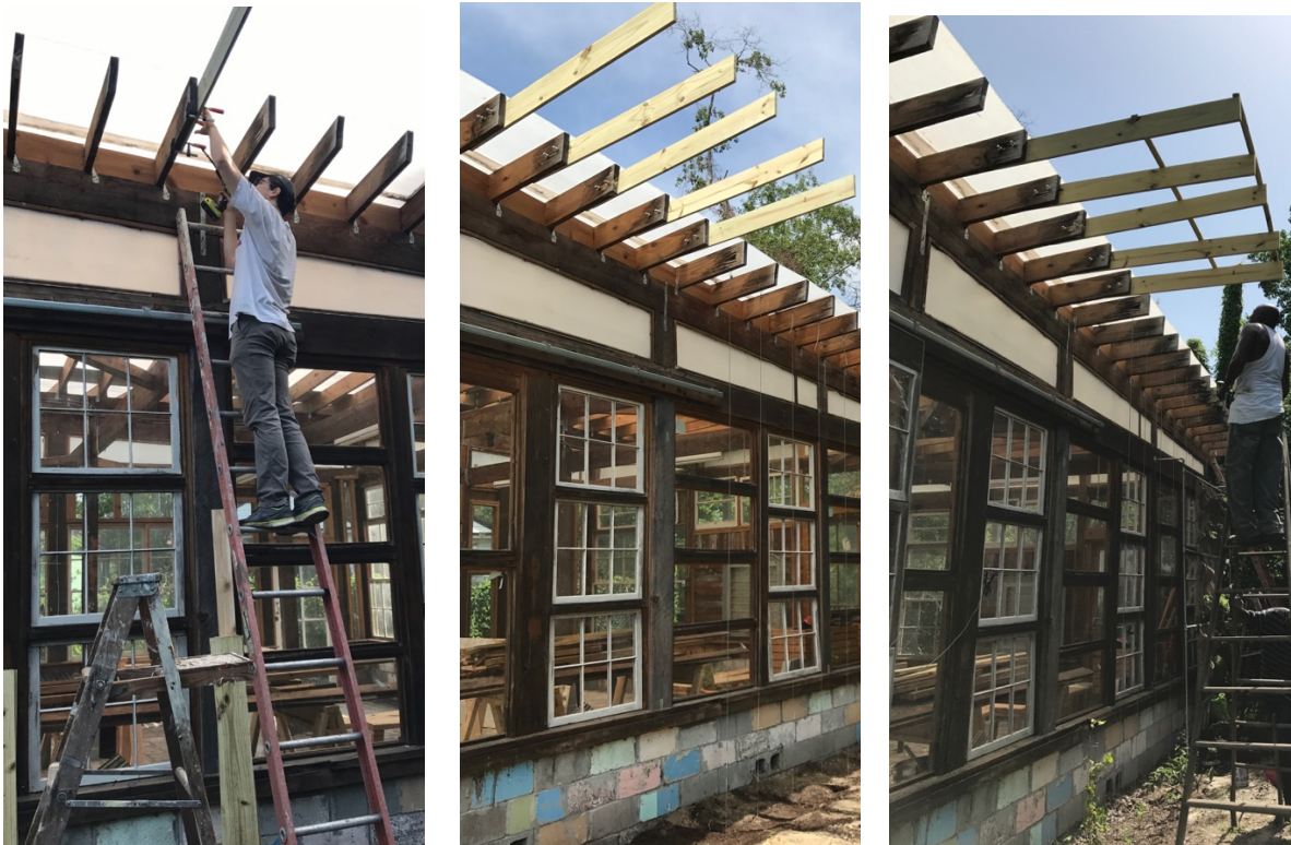
Figure 51. Overhang System Installation Process
