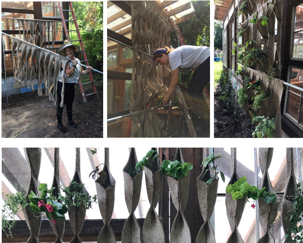
Figure 55. Pictures of Felt System Installation
