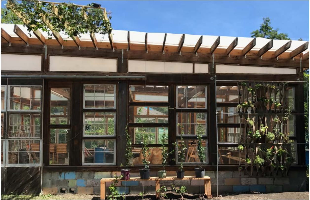
Figure 66. Final Green Façade System Installation at E. 34 Greenhouse
